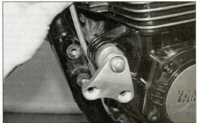
5.21b Slip the hydraulic hose out from between the engine and frame
